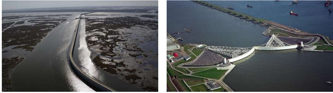
Figure 4-31: Protection measures through the construction of fixed and mobile barriers (left image, The Surge Barrier in Louisiana, New Orleans, USA. Right image, the Maeslant Kering Barrier, The Netherlands).
