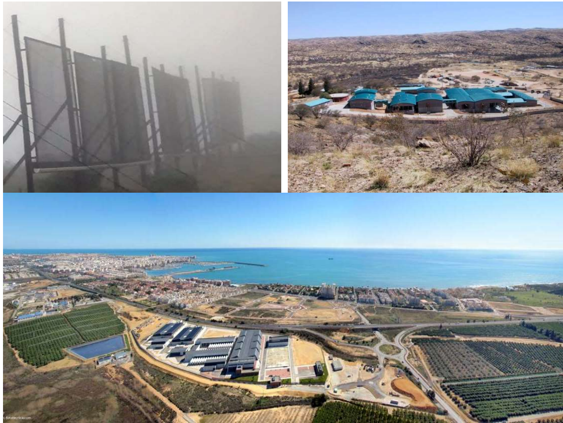
Figure 4-19: Unconventional resources are essential in areas where water scarcity has become structural or necessary to release other water resources for environmental purposes. Fog water harvesting can provide between 2 to 10 l/m 2 per day (top left image - fog harvesting meshes in Chile-). Water reuse treatments make it possible to reuse the resource mainly for agriculture. However, in some countries, such as Namibia, it is used for water supply (top right image - water reuse plant in New Goreangab, Namibia.). Desalination by reverse osmosis has grown exponentially over the last few decades, mainly due to the drastic reduction in energy consumption (lower image - Torrevieja desalination plant -240,000 m 3 /day-, Spain-).
