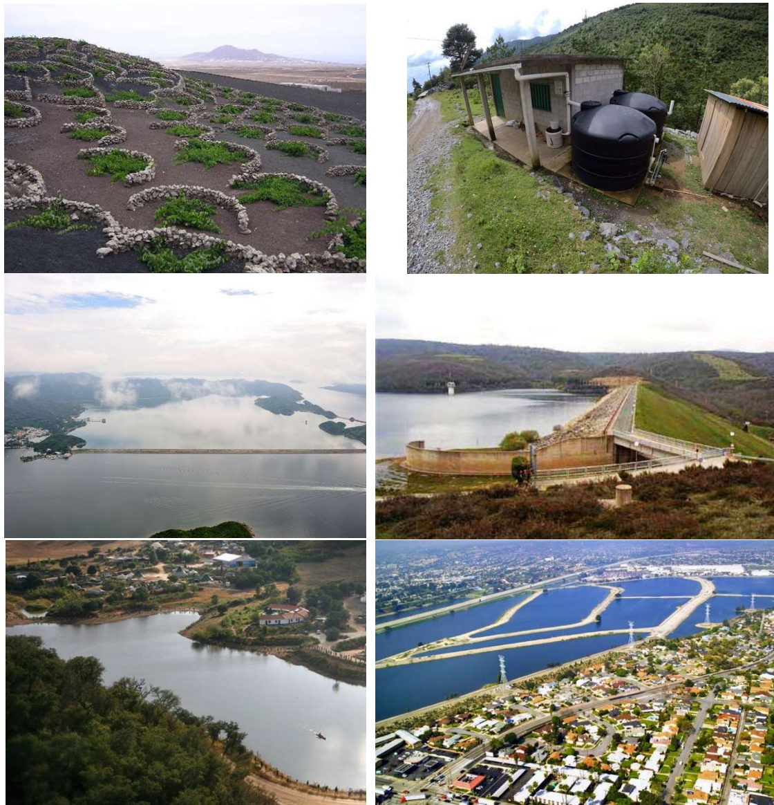
Figure 4-18: Climate change scenarios predict an increase in the temporal, spatial, and intensity variability of precipitation. Given this situation, there is a need to increase water harvesting and storage. This can be done through rainwater harvesting and storage (top left image -water retention with semicircular banks- and right image -rainwater harvesting-), reservoirs (middle left image -Plover Cove coastal reservoir in Hong Kong- and right image -Uzquiza dam in Spain-), creation of water retention areas (lower left image -water retention landscape of Tamera, Portugal-) and aquifer recharge (lower right image - aquifer recharge pond system in California-, USA).
