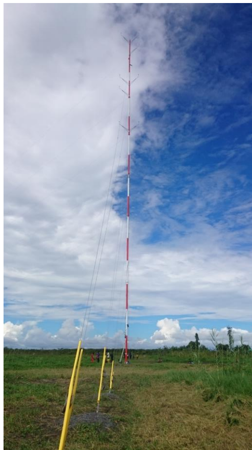
Figure 3: The NRG 60m mast installed at Kasomalunga in Luapula.
